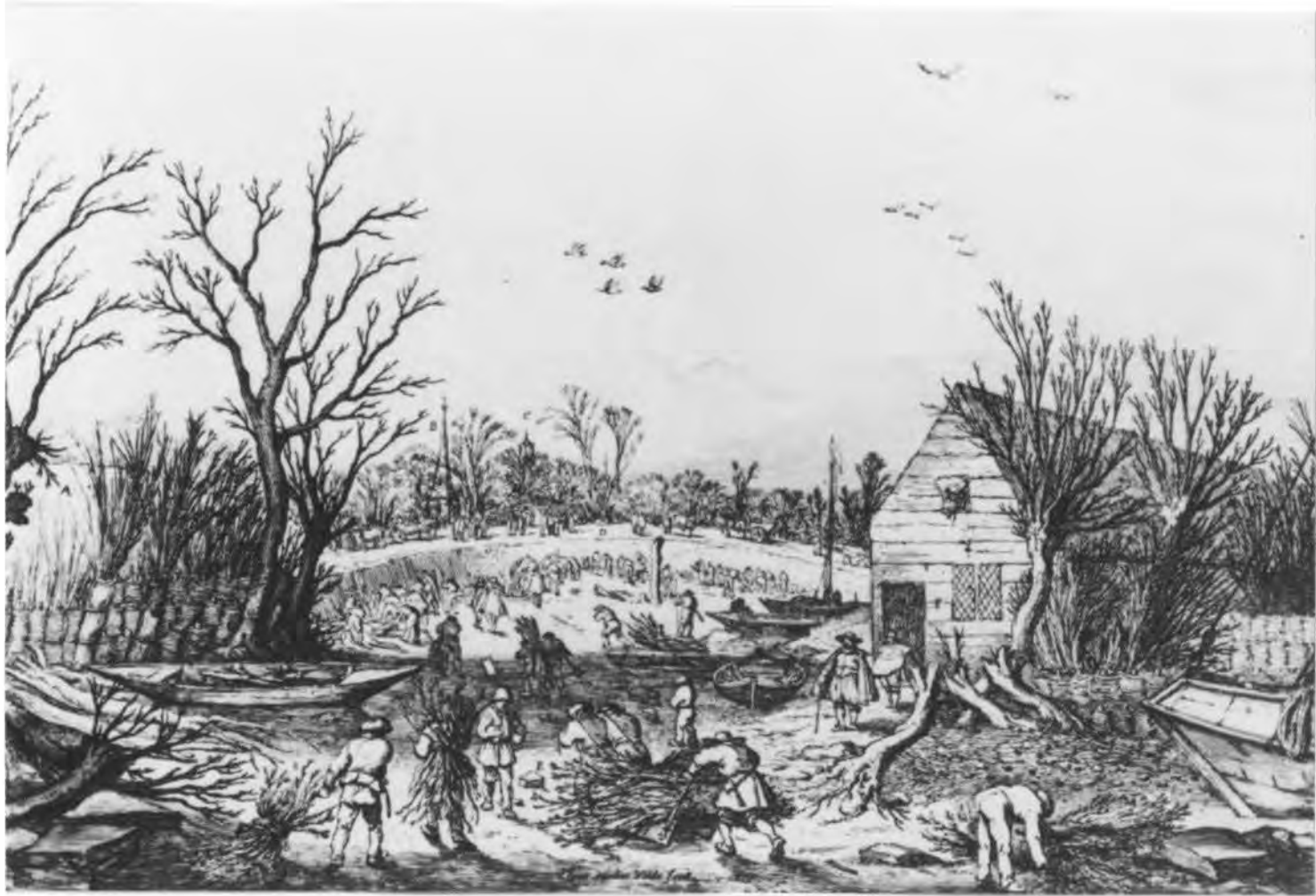
Dutch farmers work feverishly to repair the dikes before next year's rains. Willow branches - called rijs - are hauled in to form the underpinnings. In the Bommelerwaard, farmers like Ott van Tuyl not only repaired their assigned dike sections, but participated in a major overhaul of the Meidijk [Drawing by E. van de Velde, in H. van Heiningen: "Dijken en Dijkdoorbraken," Den Haag, 1978, pg. 11].
